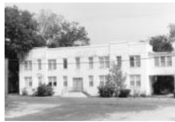
Mullins Commercial Historic District (S10817734008)
