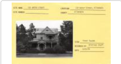
110 Water Street (S108042001300146)
