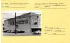
The Corner Factory Outlet (S108042001400205)
