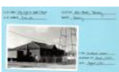
City Light & Water Plant (S108042001400180)
