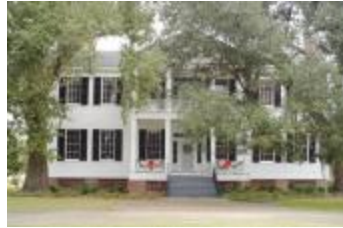
Davis House (S10817714002)
