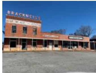
Bracknell's Store Complex (S10817733023)
