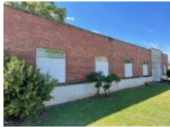
McCormick County Office Building (S10817733022)
