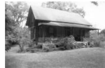
Socastee Historic District (S10817726024)
