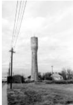
Belton Standpipe (S10817704006)
