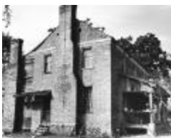
Means House (S10817744006) Object identifier: S10817744006 Name: Means House
