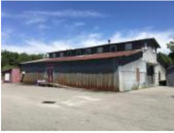
Storage building (S108042000003875)
