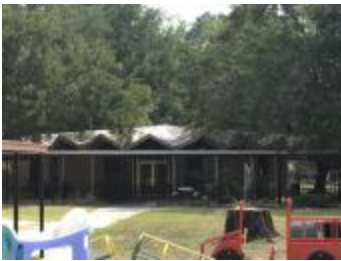
Private school building (S108042000003931)
