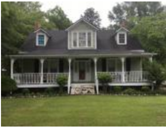
Reid House (S108042000003543)
