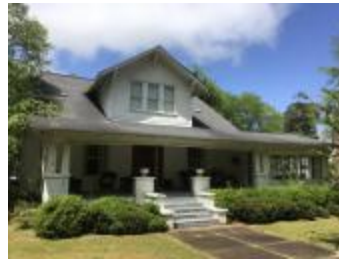
Funderburk House (S108042000003665)
