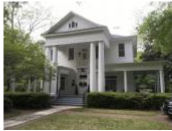
Harrall-Godfrey-Spruill House (S108042000003612)
