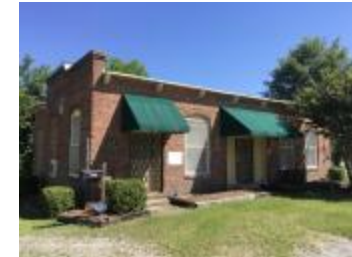
CP and L Building/ Cheraw Electric Generator (S108042000003758)
