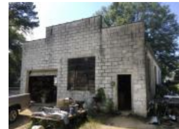
Commercial garage (S10804200003838)
