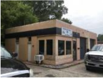
Gas station (S108042000003935)
