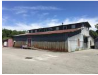
Storage building (S108042000003876)
