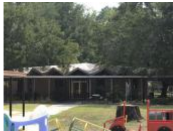
Private school building (S108042000003932)
