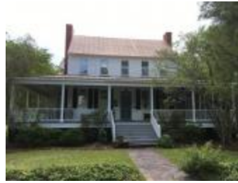
Coit-Poston House (S108042000003625)
