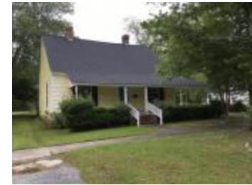
Bundy-Davis House (S108042000003522)
