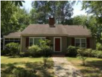
Kornegay House (S108042000003447)
