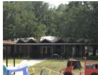
Private school building (S108042000003933)
