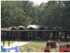
Private school building (S108042000003933)
