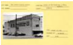
The Corner Factory Outlet (S108042001400205)
