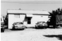
Blue Block Building (105.02)
