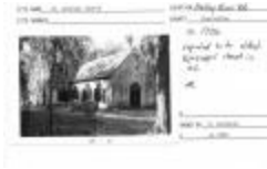
St. Andrews Church (S108042002300206)
